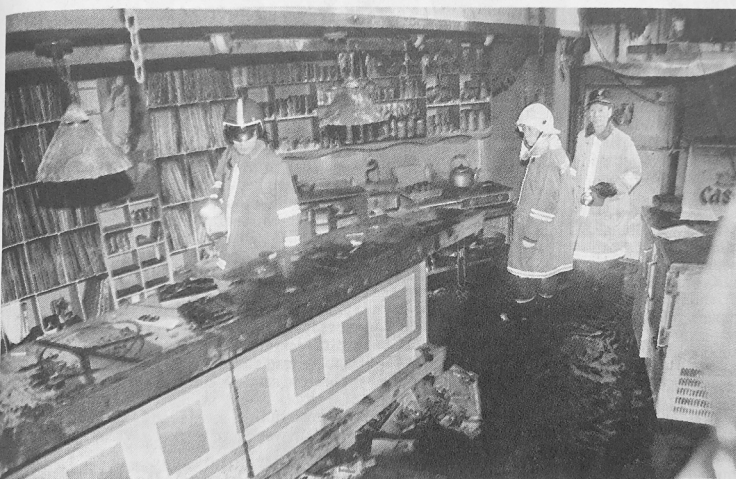
Firefighters Monday examine the interior of the basement cafe, "Rolling Stones," which was completely gutted by an evening fire Sunday. Eleven people died and three others were severely injured in the blaze of yet unknown cause.
