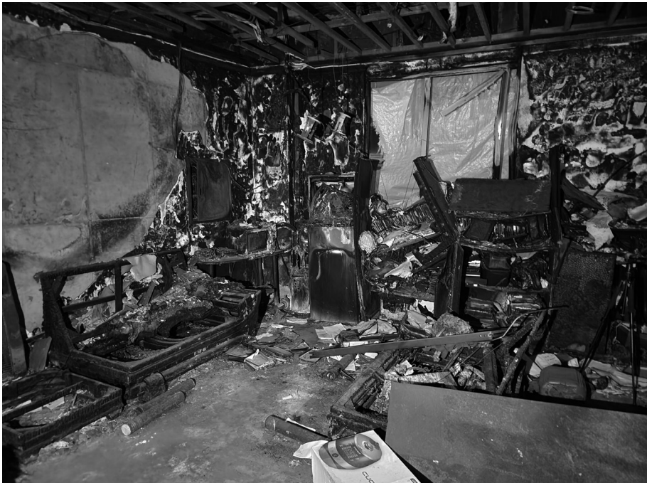
Looking back in the opposite direction toward the window I'd peered in through, you can see that wall covered in fire damage. It's my understanding that these signs indicate the fire started somewhere over there.
