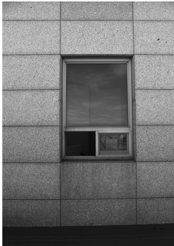
The only way off the roof is through this tiny window, 20240928. Dunbar roll is needed.
