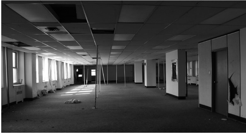
Probably the most serious urban exploration I ever did in Edmonton, way back in 2008. And it was done with permission.
