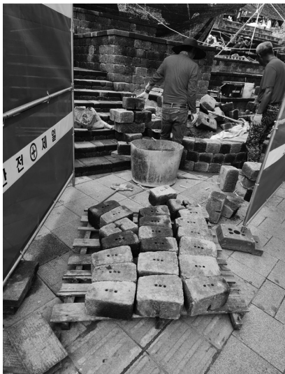
Workers carry stone bricks in, 20250826.
