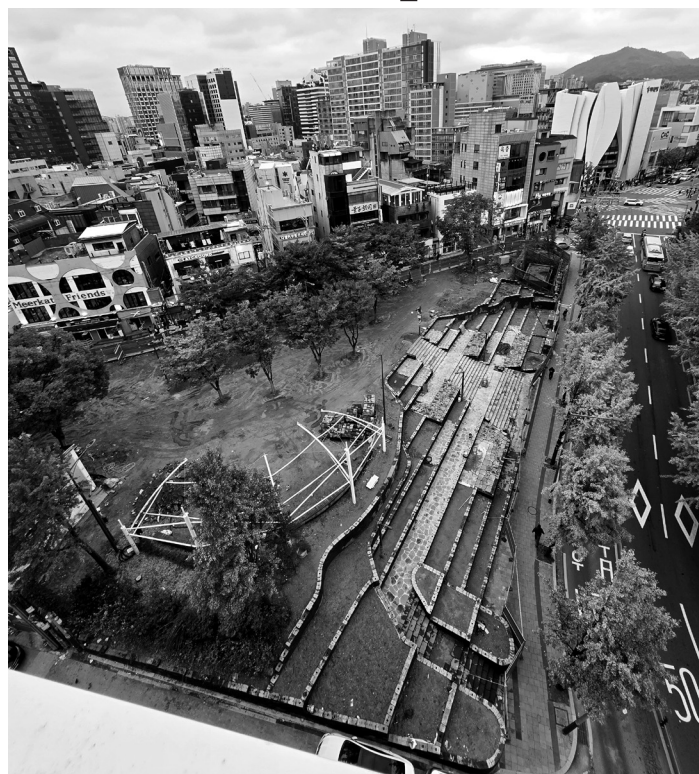
An overhead view of work being done on Hongdae Playground, 20251018.
